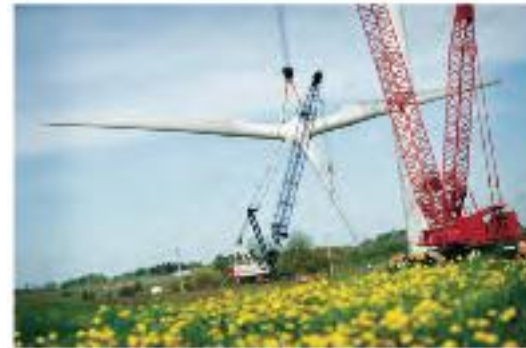
Top: Engine for waste biogas energy project on Gundersen's Onalaska Campus (May 2012). Bottom: Wind turbine energy project in Cashton, Wisconsin (May 2012). Photos: Gundersen Lutheran.
